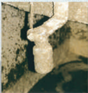
KAB 10 COVERED WITH MATERIAL
