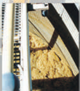
KAB 10 WORKING ON FOAM
